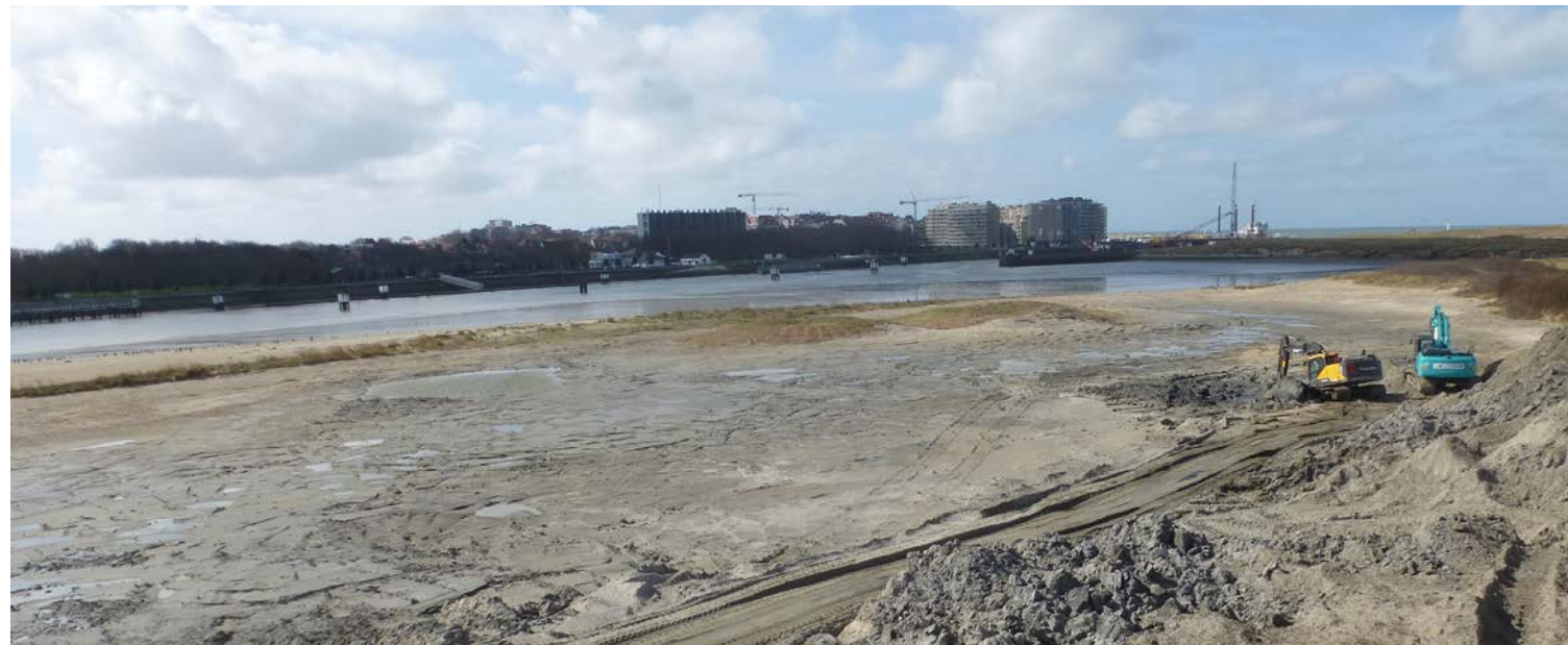
"Outside Life": Removal of dredging sludge dump at the Yzer estuary to restore tidal mud flats (1130) and salt marsh (1310-1330) ©Stijn De Ruyter
